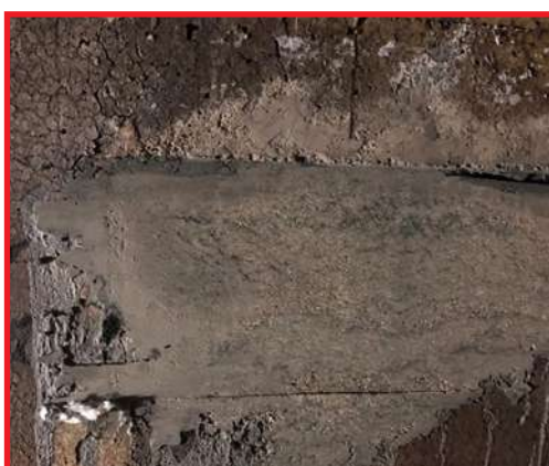
REPAIRS COMPLETED ON THE WALL
